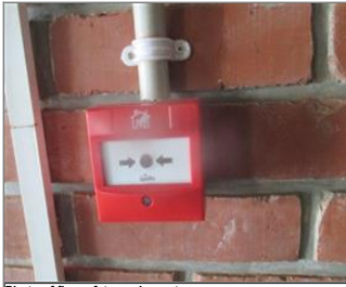
Photo of fire safety equipment Fire call point.jpg
