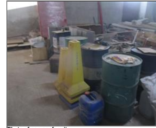
Photo of non-conformity Chemical without MSDS label and secondary containment.jpg
